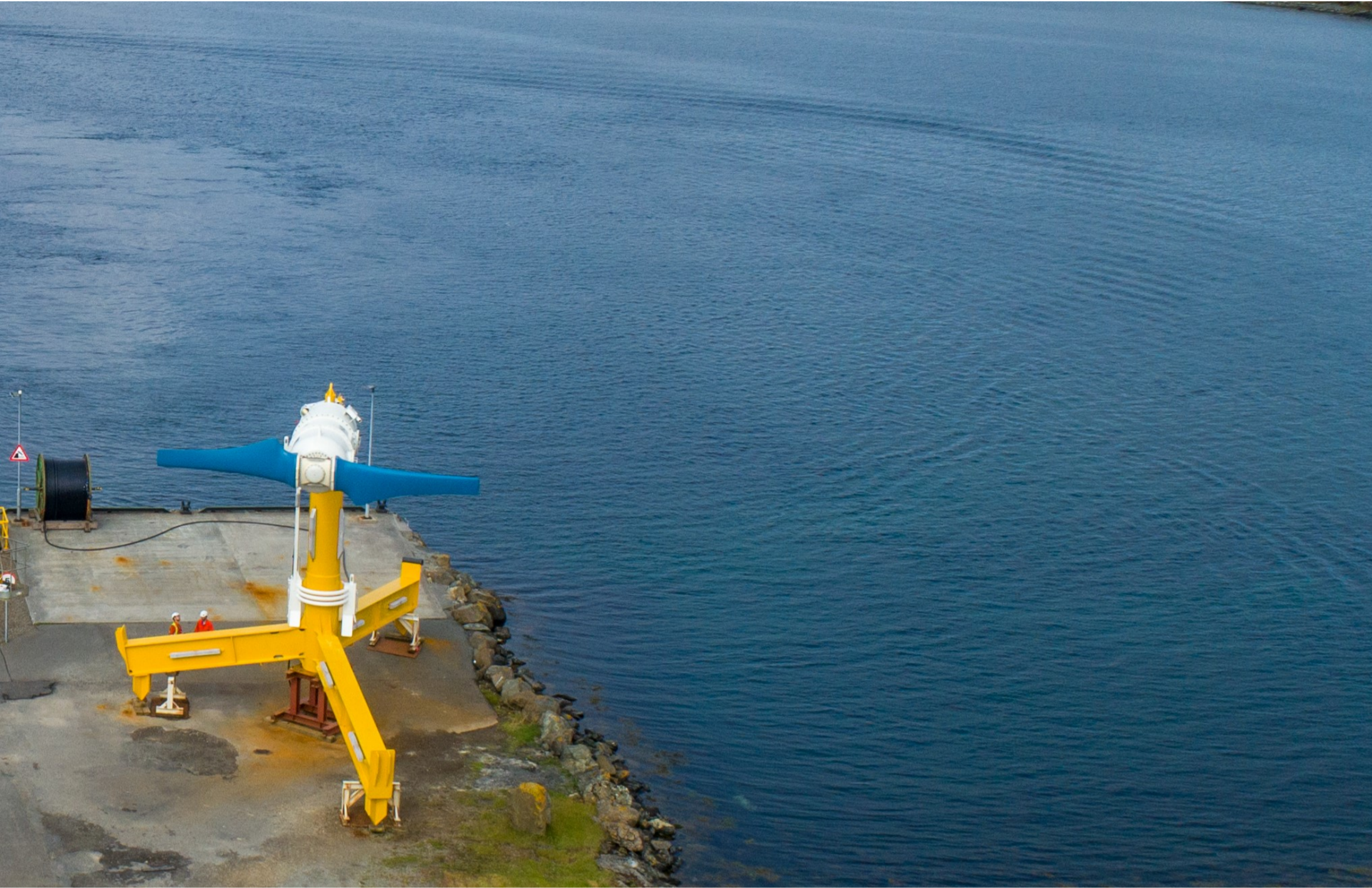
T4 turbine prior to offshore deployment in Shetland, Scotland
